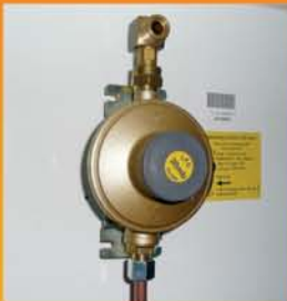
Replaced regulator using the existing compression nut and olive. Unit shown has an optional right angle adaptor (01-1677-300) fitted on top due to height restriction.
